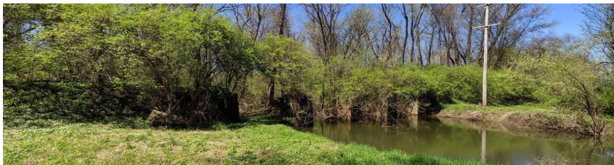
The canal grade and Pigeon Creek Aqueduct remnants (photo taken May 2019)
