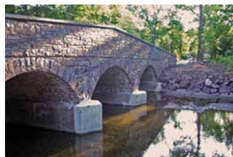
Fagelysville Road Bridge
