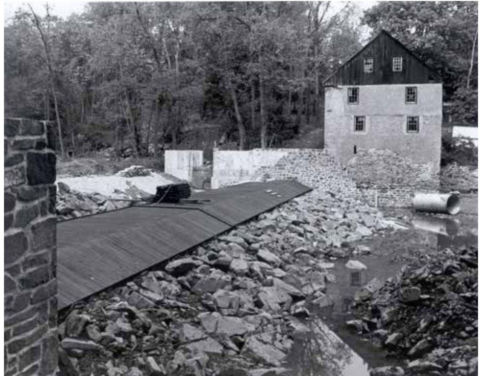
Sunrise Mill Dam under construction.
