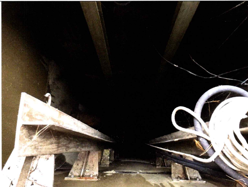
2 Pump Station #7 – Wet Well Interior.
