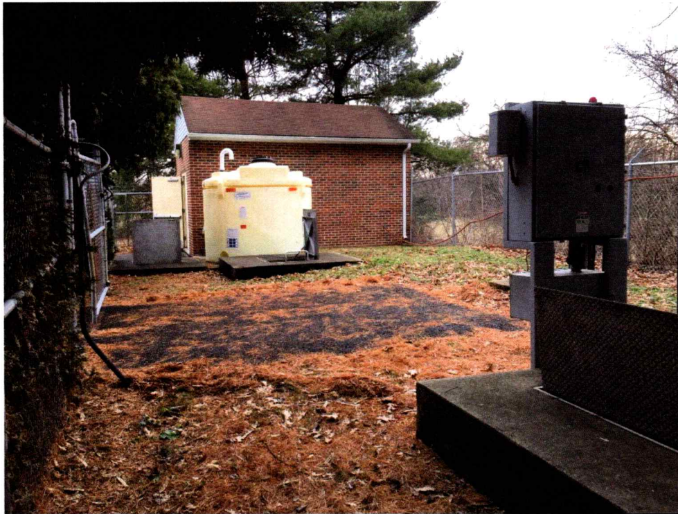
1 Pump Station #7 – Overall Site.
