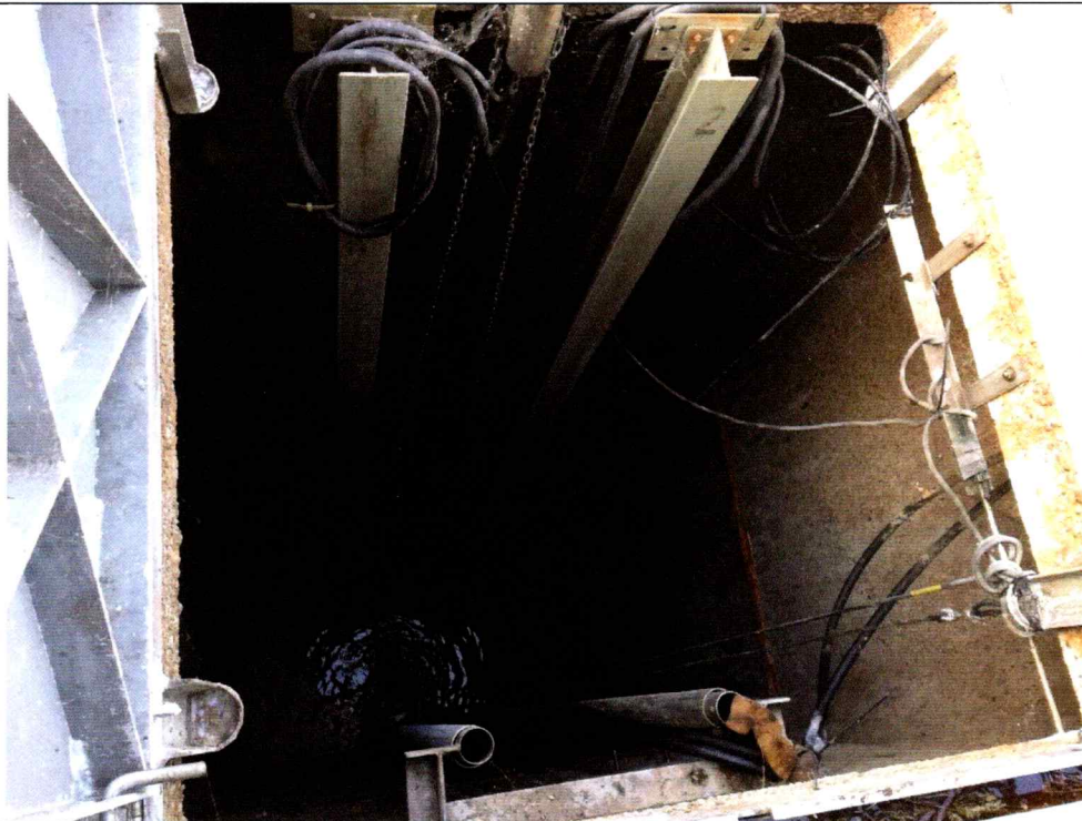
2 Pump Station #2 – Wet Well Interior.
