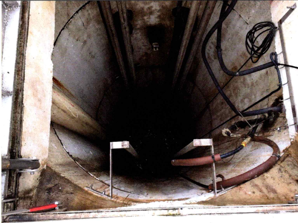
2 Pump Station #12 – Wet Well Interior.
