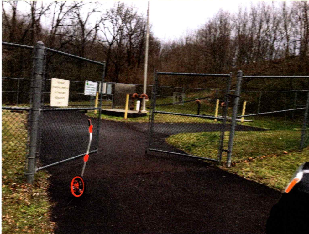
1 Pump Station #16 – Overall Site.
