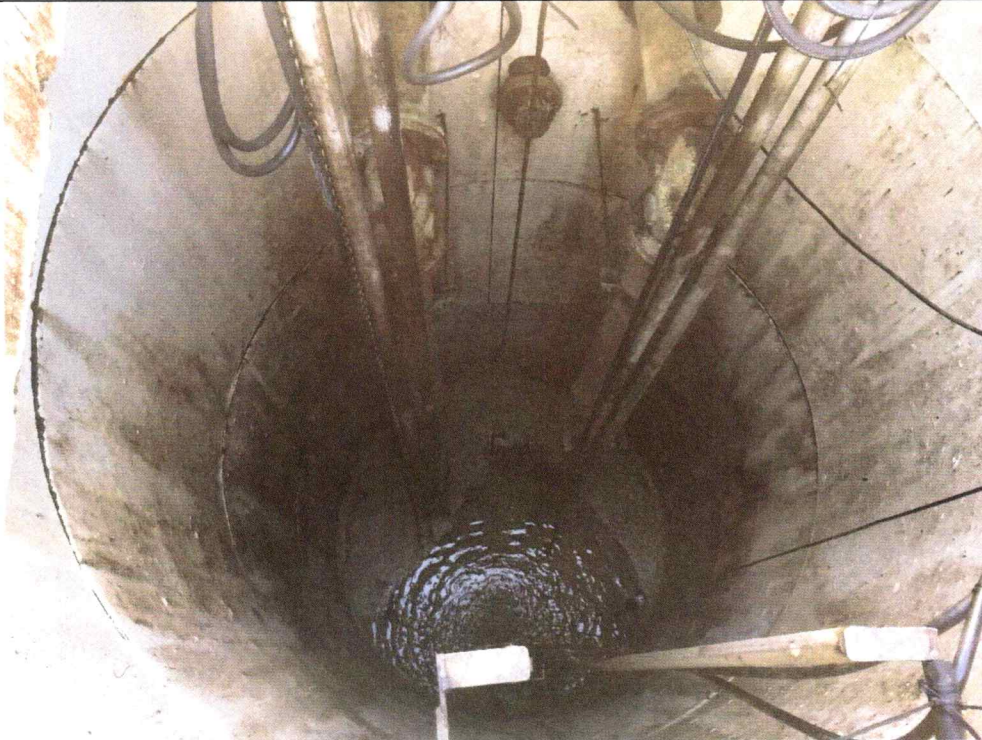
2 Pump Station #10 – Wet Well Interior.
