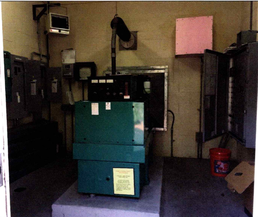
4 Pump Station #13 – Building Interior.
