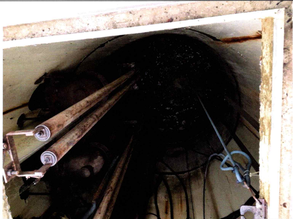
2 Pump Station #17 – Wet Well Interior.
