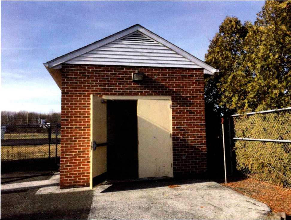
3 Pump Station #2 – Building Exterior.
