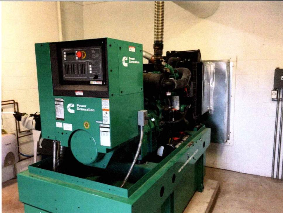
4 Pump Station #20 – Building Interior.
