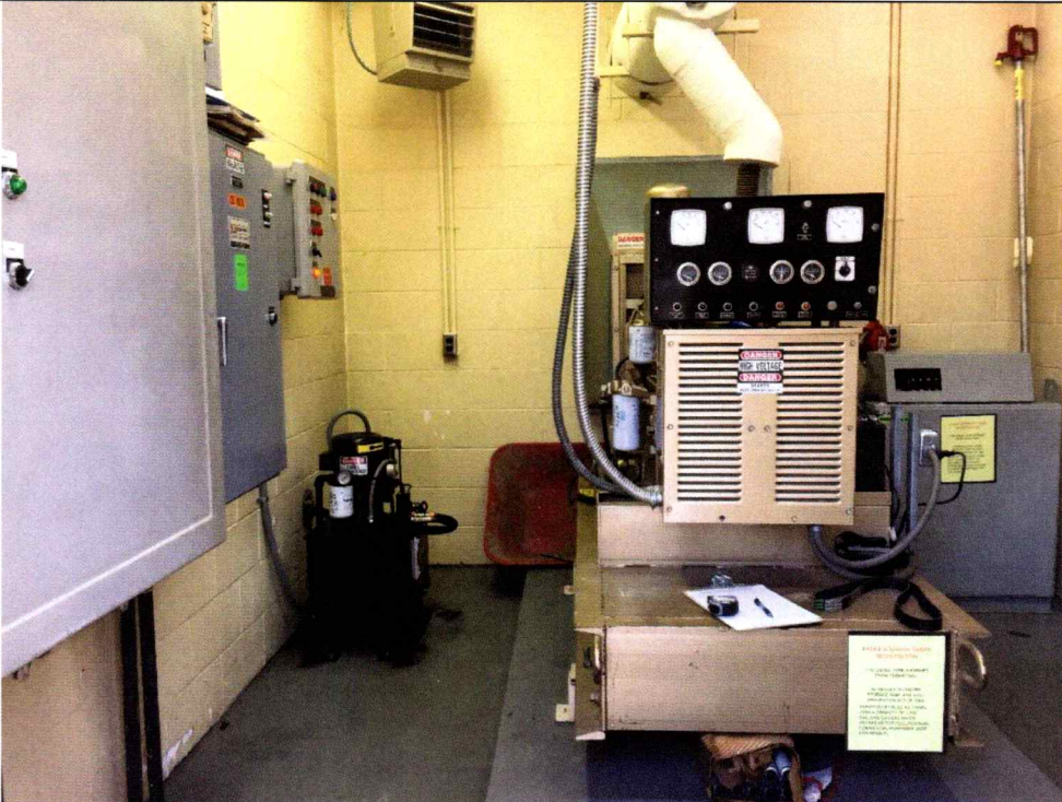
4 Pump Station #2 – Building Interior.
