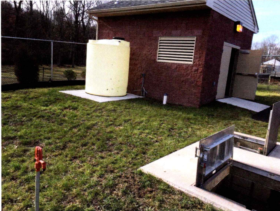
3 Pump Station #20 – Building Exterior.
