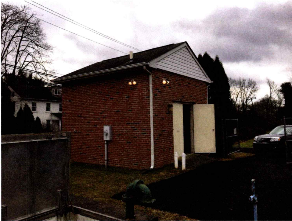
3 Pump Station #12 – Building Exterior
