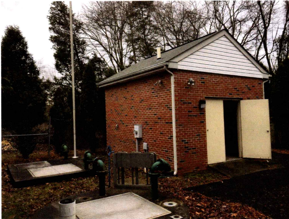
3 Pump Station #14 – Building Exterior.
