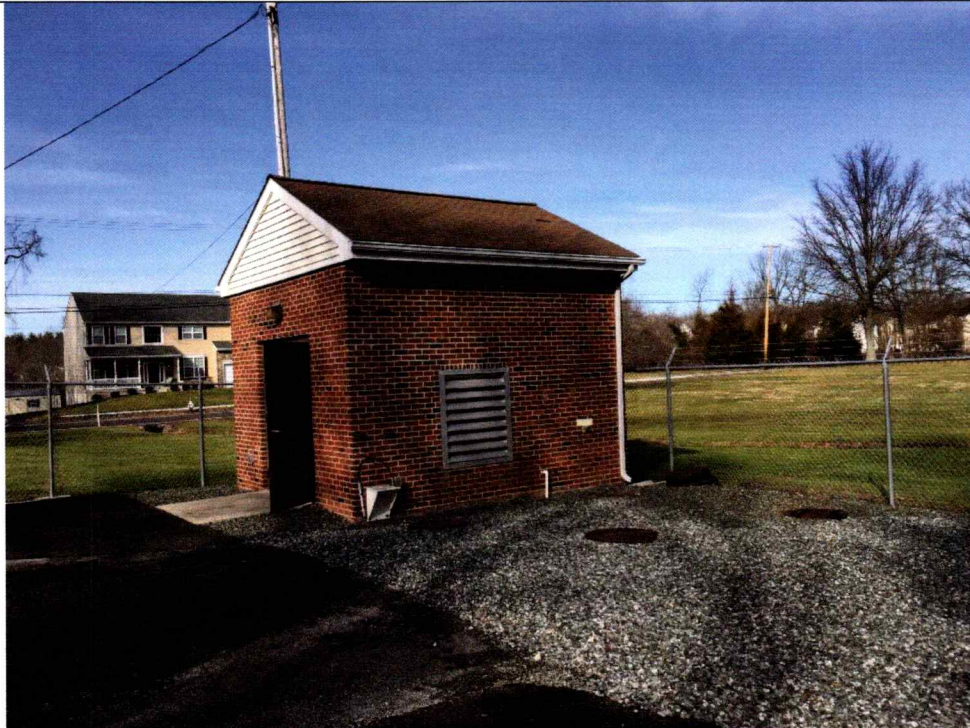
2 Pump Station #9 – Building Exterior.
