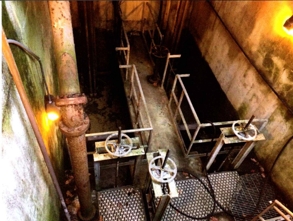
3 Pump Station #5 – Wet Well Interior.
