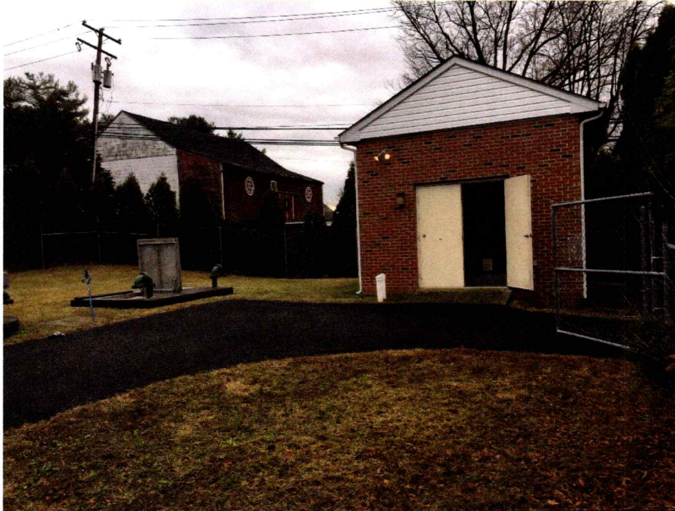
1 Pump Station #12 – Overall Site.
