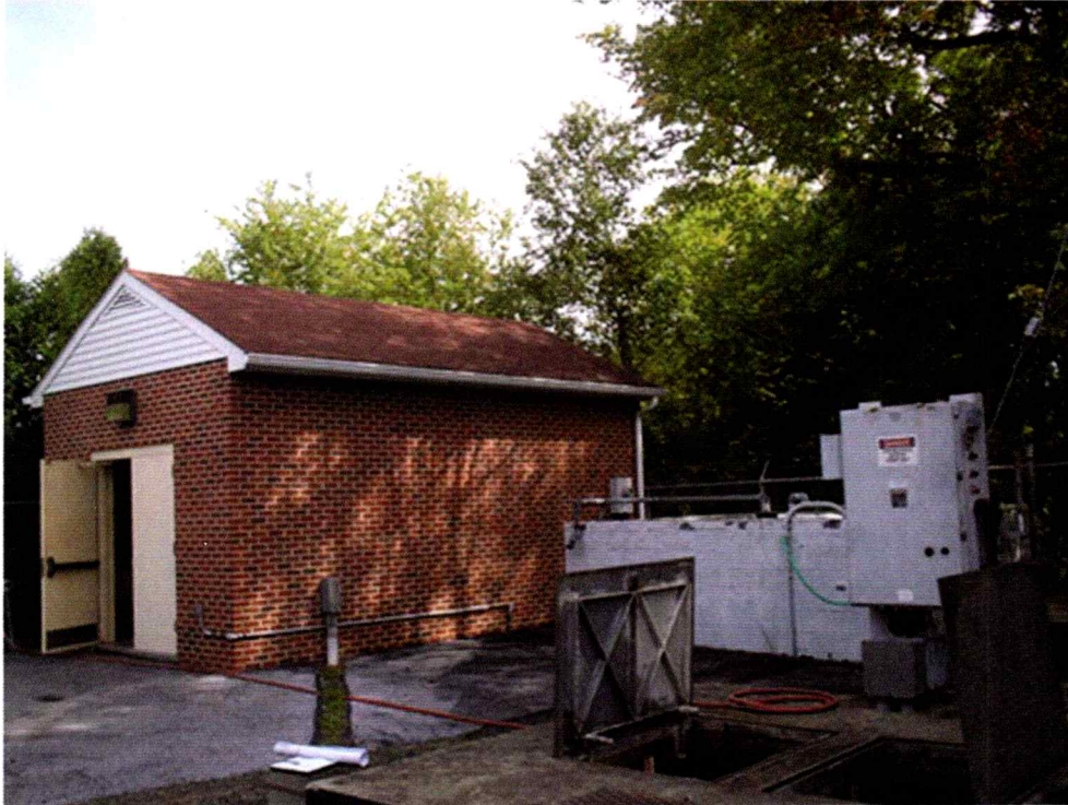
1 Pump Station #3 – Overall Site.
