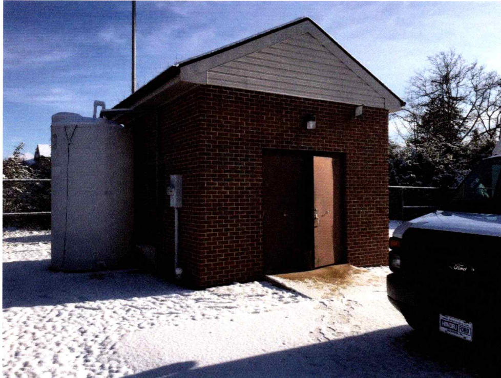
3 Pump Station #10 – Building Exterior.
