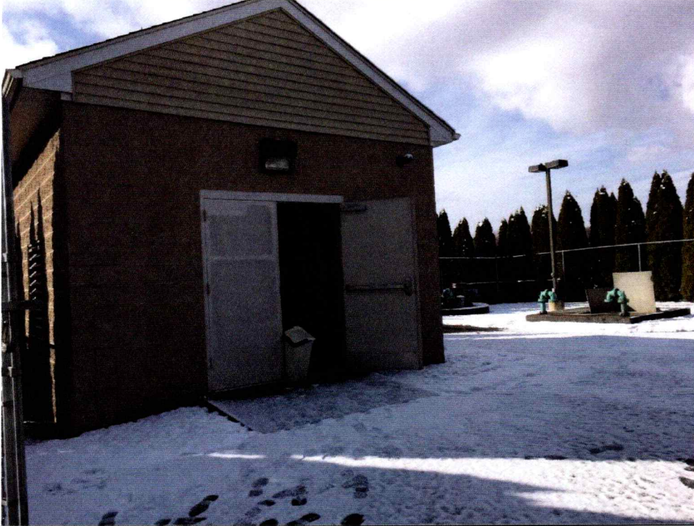
1 Pump Station #3 – Overall Site.
