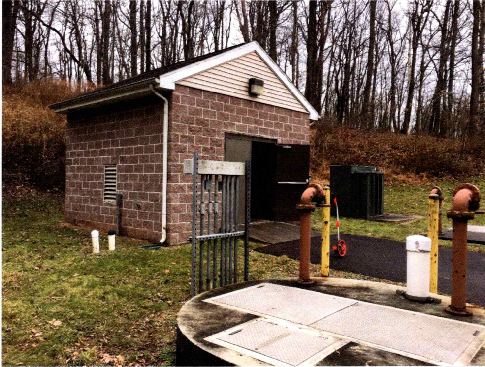
1 Pump Station #17 – Overall Site.
