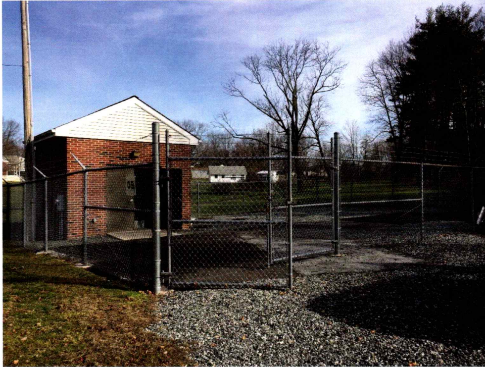
1 Pump Station #9 – Overall Site.
