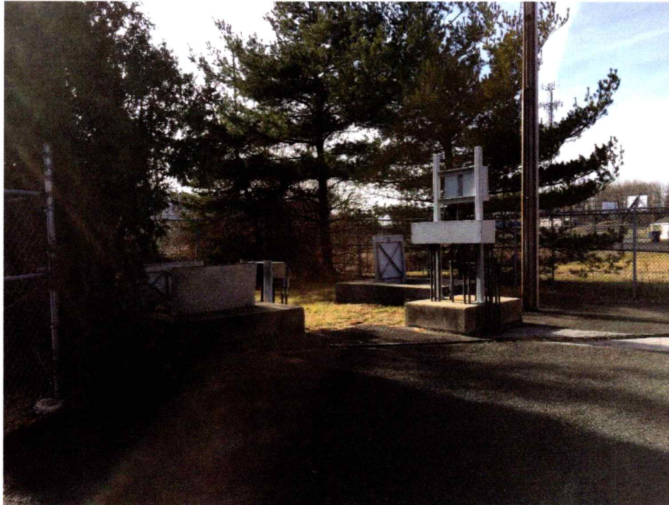
1 Pump Station #2 – Overall Site.
