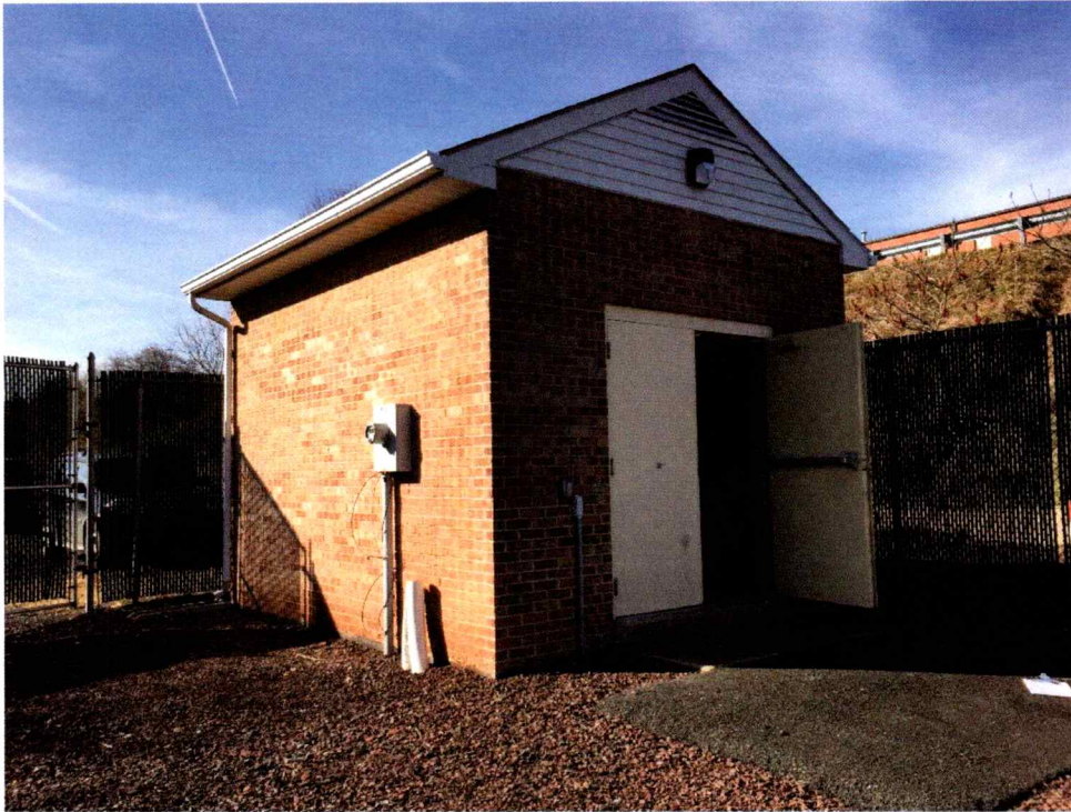
3 Pump Station #1 – Building Exterior.
