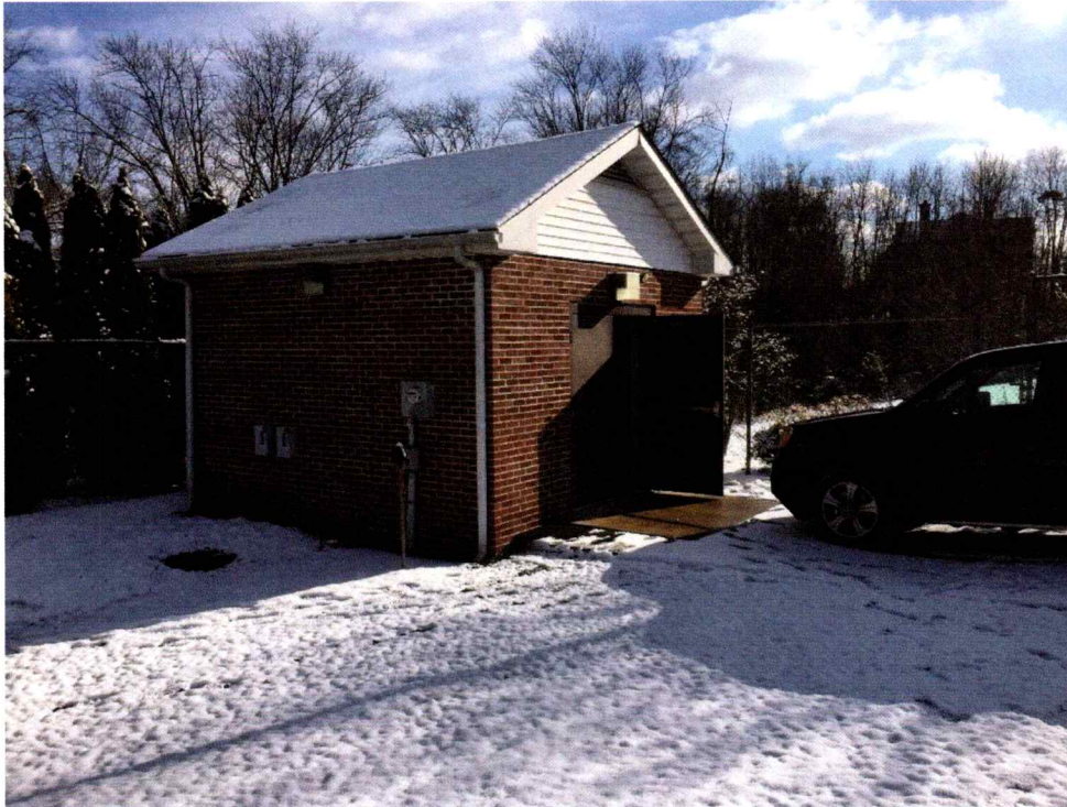
3 Pump Station #15 – Building Exterior.
