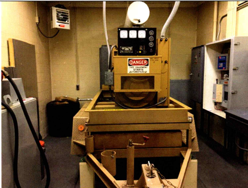
4 Pump Station #3 – Building Interior.
