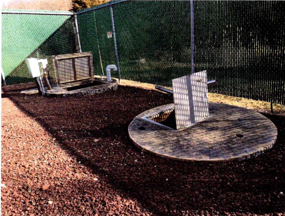
1 Pump Station #1 – Wet Well and valve chamber
