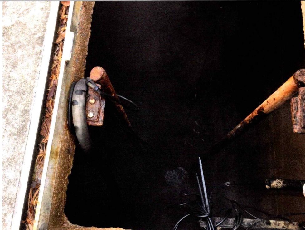
2 Pump Station #3 – Wet Well Interior.
