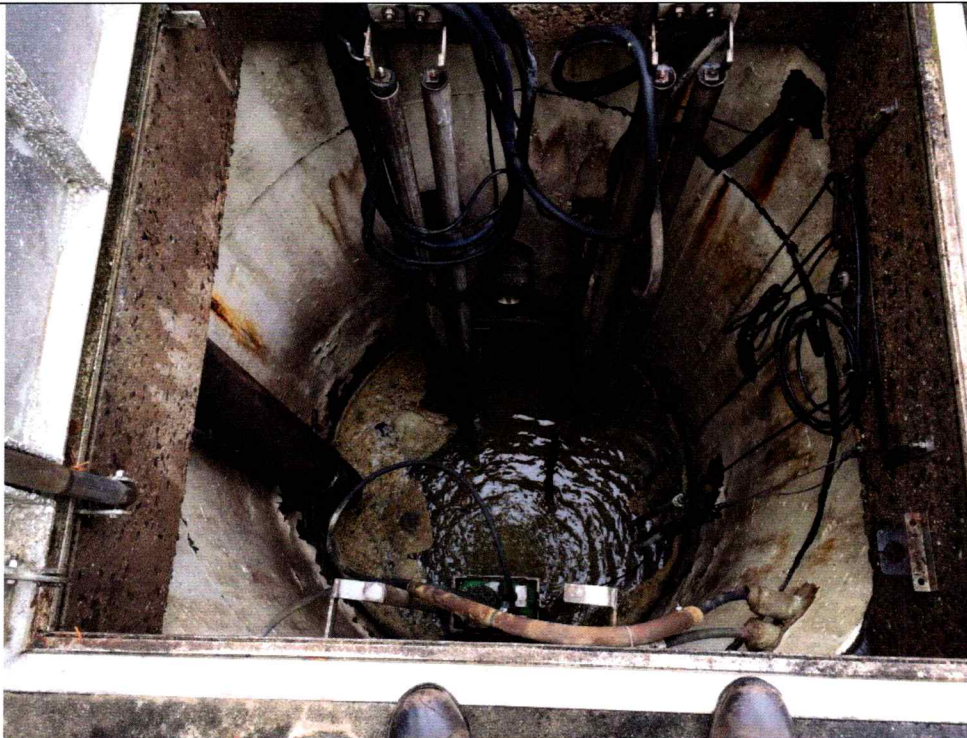
2 Pump Station #14 – Wet Well Interior.
