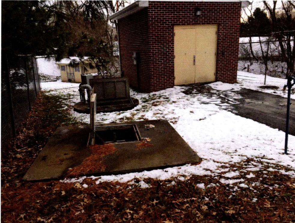
1 Pump Station #4 – Overall Site.
