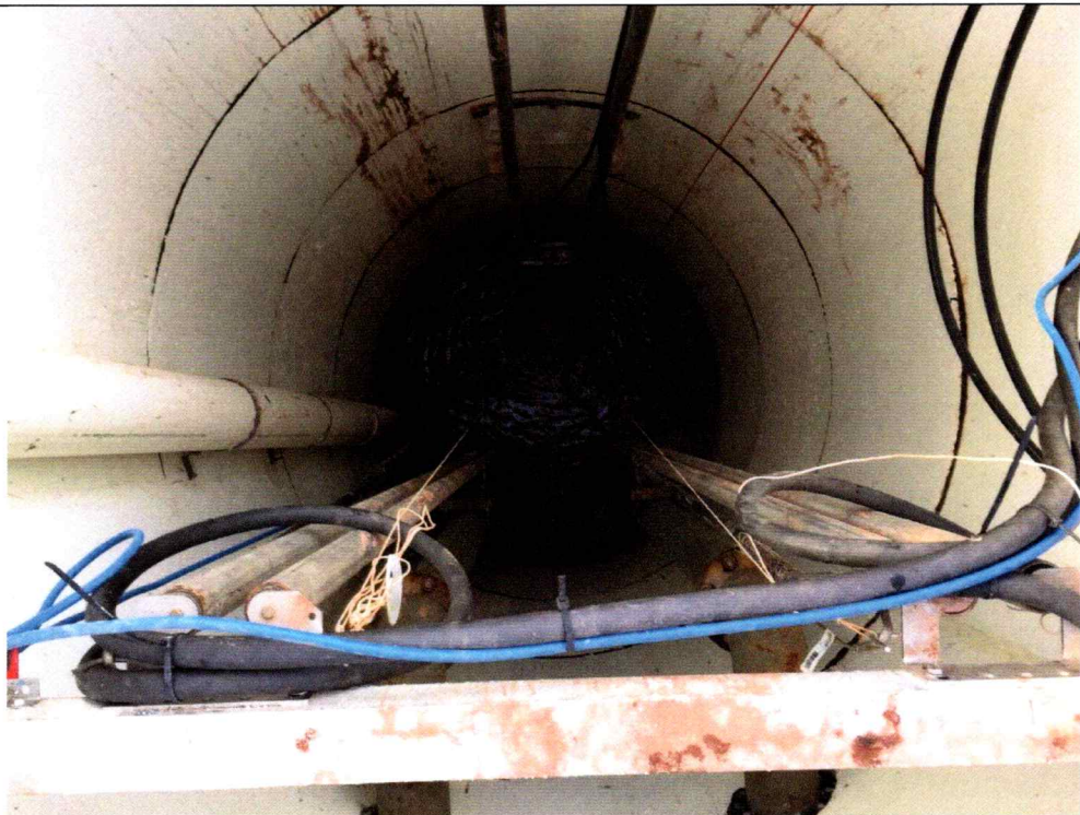
2 Pump Station #20 – Wet Well Interior.
