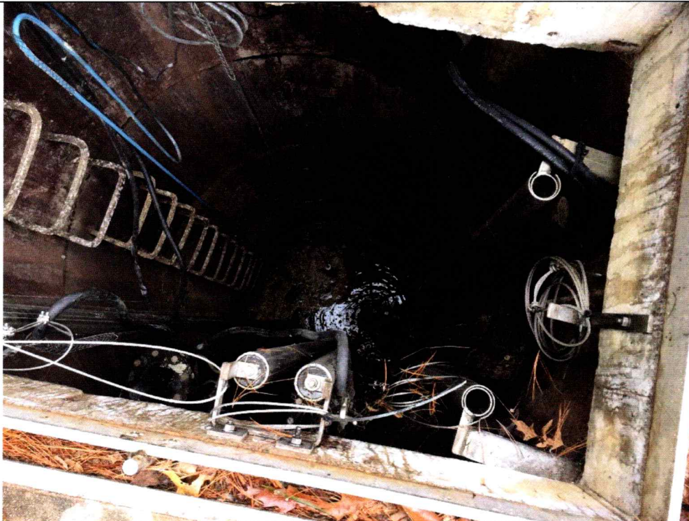
2 Pump Station #4 – Wet Well Interior.
