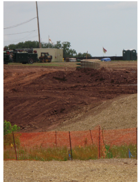
Steep slopes are especially susceptible to erosion and should be protected. The site above is adjacent to Limerick in neighboring Upper Providence Township.
