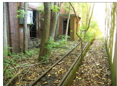
The Publicker site requires significant demolition and potentially environmental remediation.
